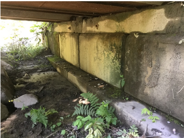
Left Bank Abutment when facing downstream
