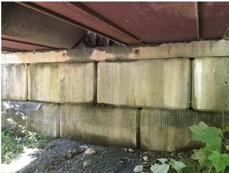
Right Bank Abutment when facing downstream
