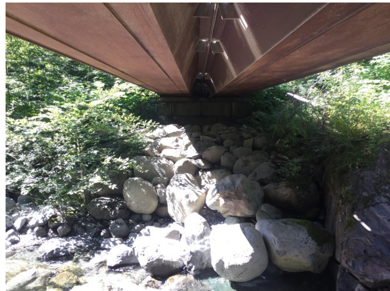
Right Bank Abutment when facing downstream
