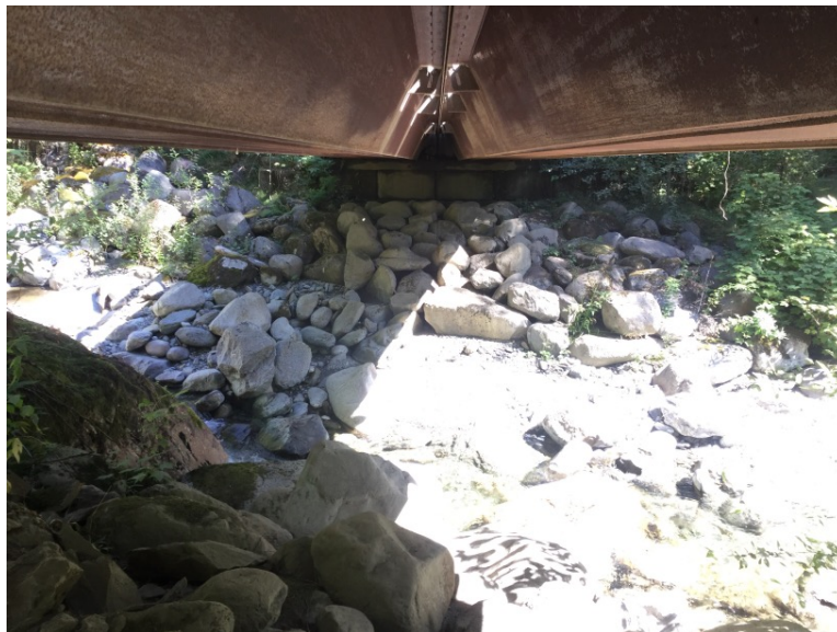
Left Bank Abutment when facing downstream
