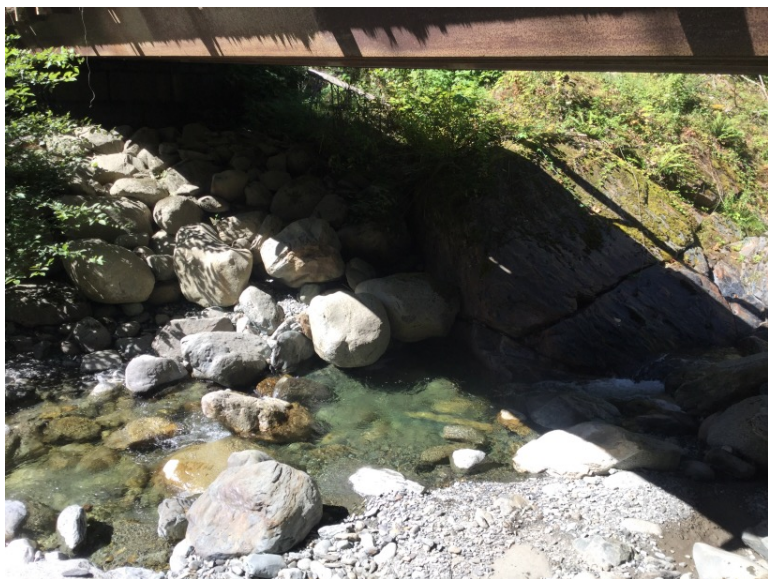
Right Bank Abutment when facing downstream
